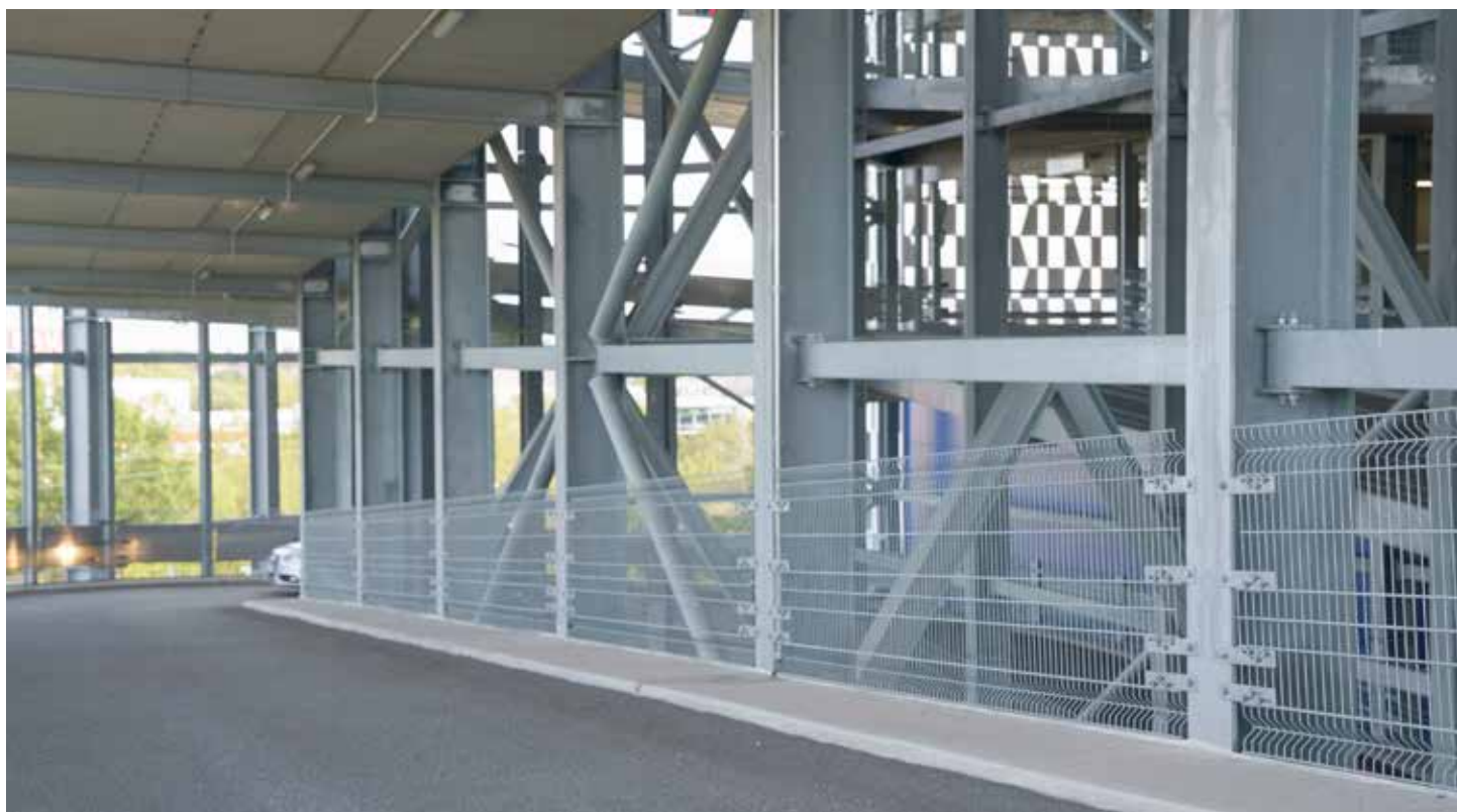
INTEGRA-pw 3.5 – multi-storey car park Furniture store
