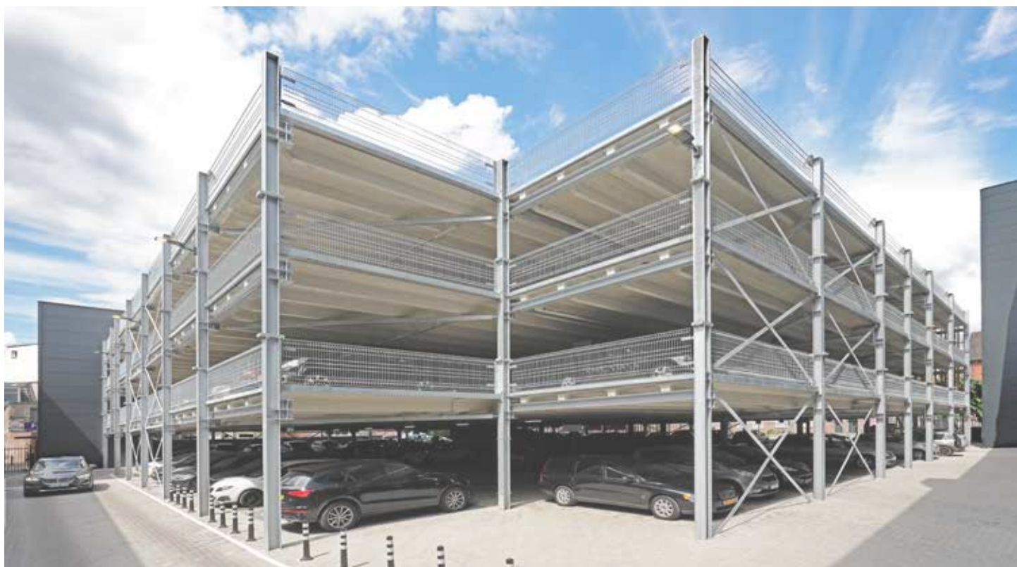
INTEGRA-pw 2.5 – Eindhoven, multi-storey car park Arsenaal
